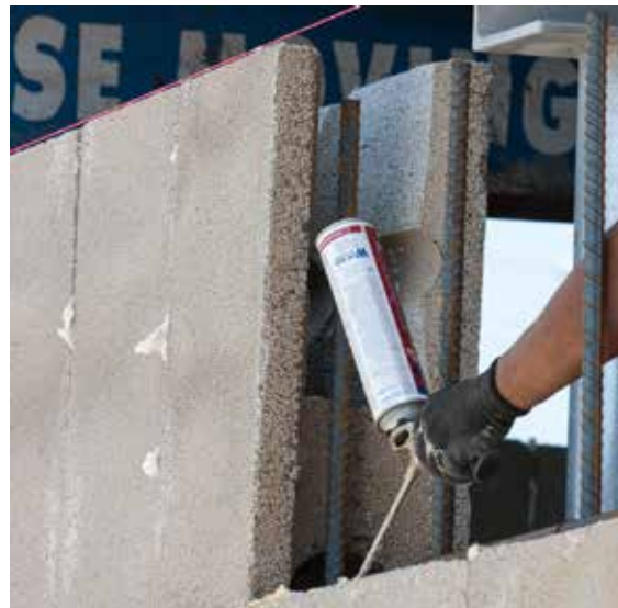
Figure 14: Bond beam cut out of Bautex Block
