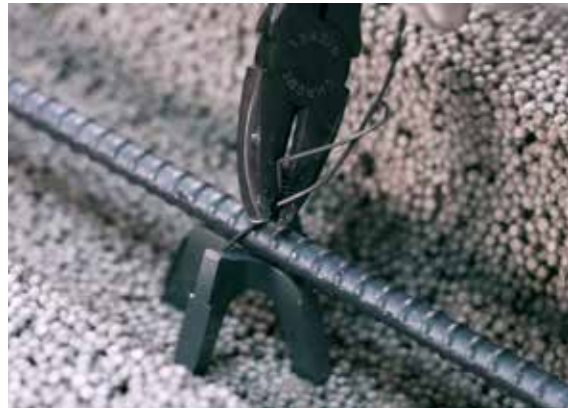
Figure 7: Tying reinforcement to rebar chair
