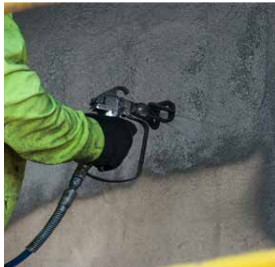
Figure 19: Application of air and moisture barrier
