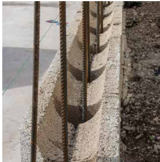
Figure 2: Laying first course of Bautex Block
