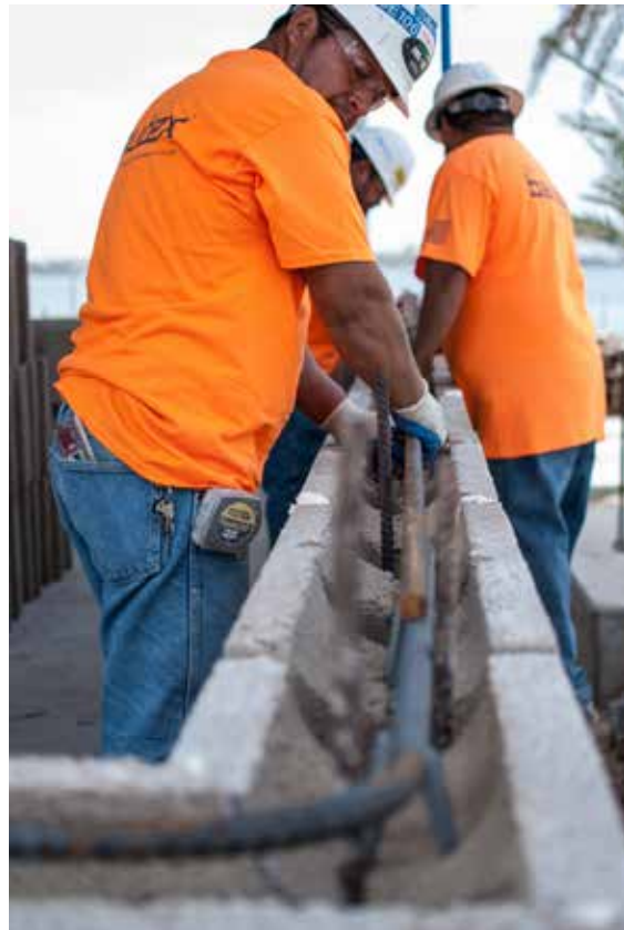
Figure 5: Placing horizontal reinforcing steel
