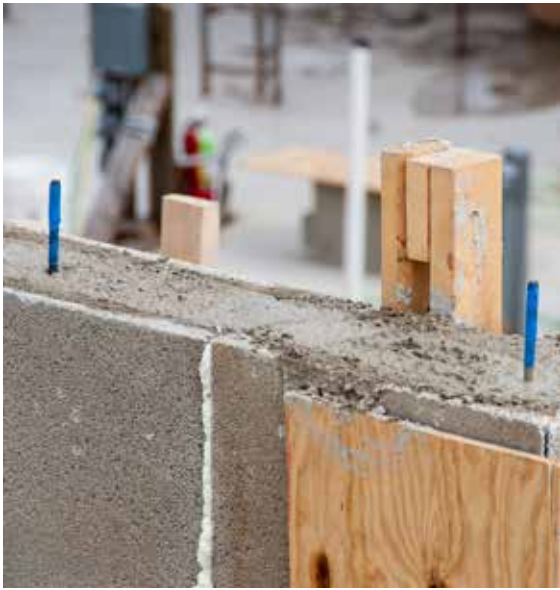
Figure 15: Wet-set J-bolts for wall top plate
