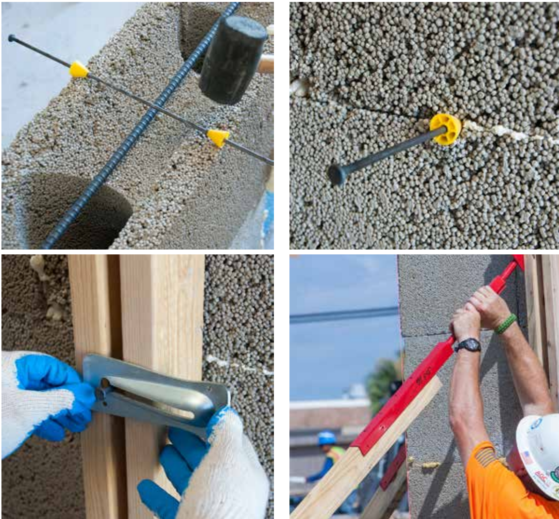
Figure 9: Installation of snap-ties, wedges and bracing
