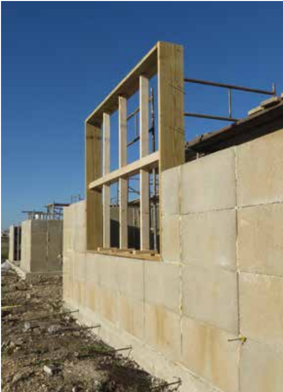
Figure 13: Stay-in-place wooden window buck
