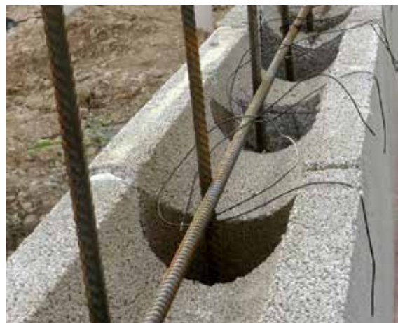
Figure 8: Wire loops for vertical reinforcement ties
